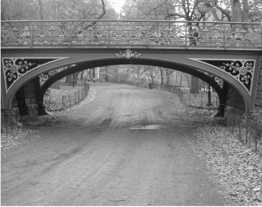
Fig. 5.47. An example of what our theory calls a compressive arch .
