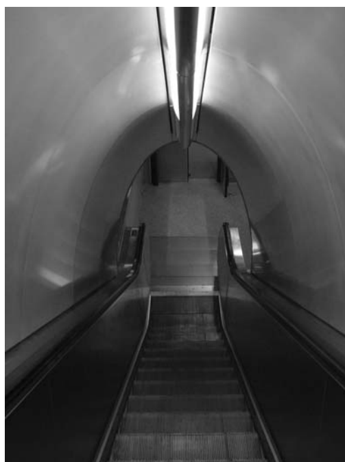
Fig. 5.46. The penetrative-arched ceiling over the same escalator.
