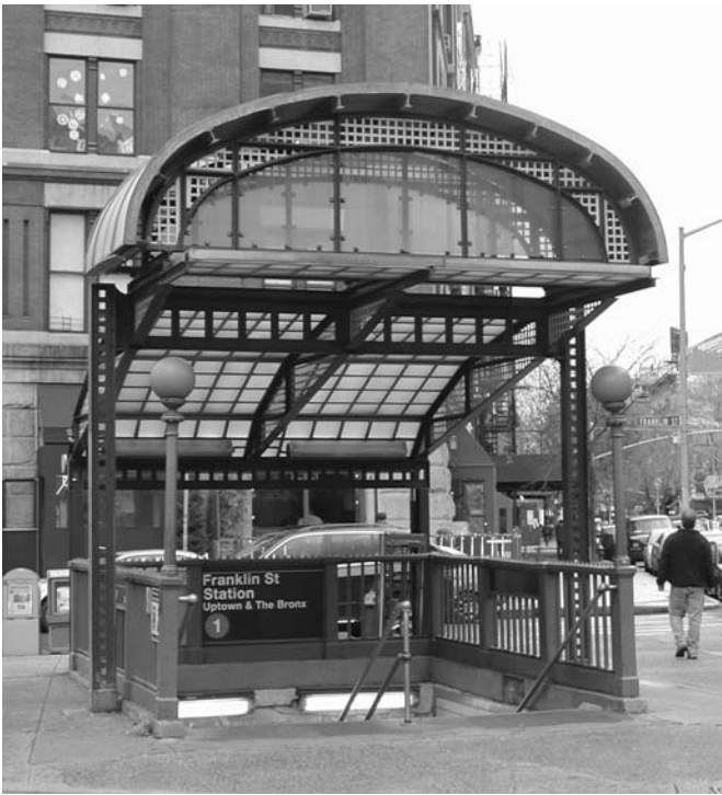
Fig. 5.20. Entrance to a subway station defined by a double-shield structure.
